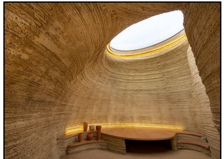
FIGURE 8d: Mario Cucinella Architects, TECLA 3D printed house (interior detail), 2021.
