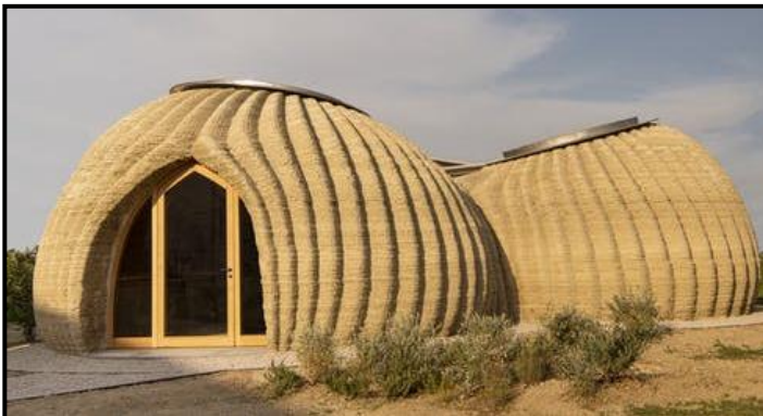
FIGURE 8c: Mario Cucinella Architects, TECLA 3D printed house , 2021. The house is constructed on site, using a mixture of clay, water, fibres from rice husks and a binder. These reusable, recyclable, carbon-neutral materials are fed into a large 3D printer that moves in a circular direction and is adaptable to any climate.
